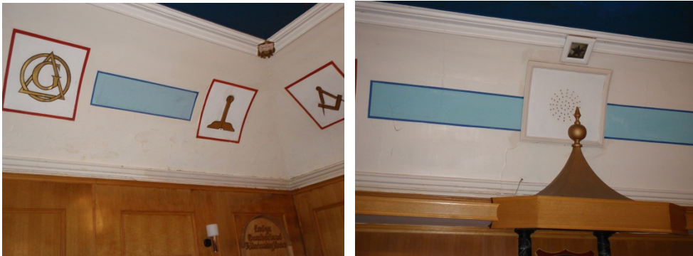
Decorative cornice and panelled walls of Temple
